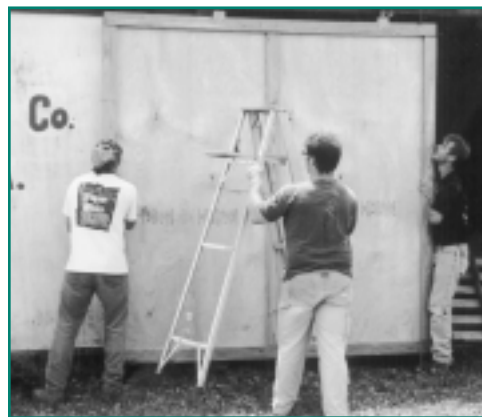
Rebuilding the carport door.
